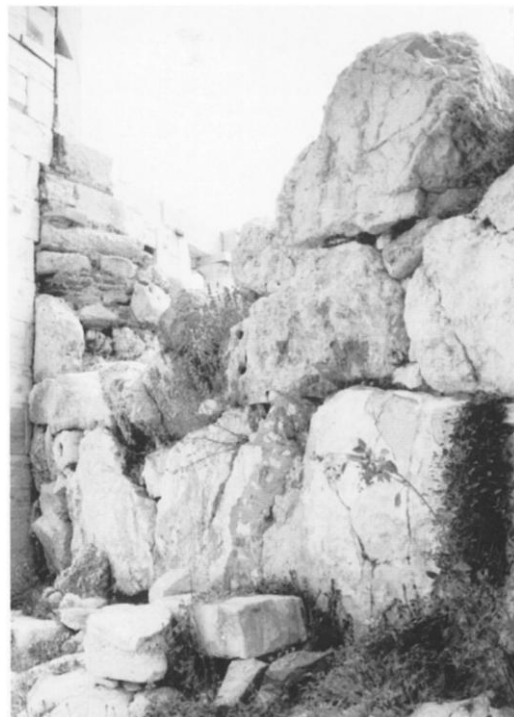
5b West Cyclopean Wall SE of SW wing of Mnesikleian Propylaea with NE corner of SW wing along left side
